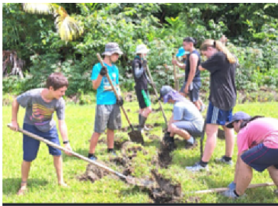
Digging ditches across the airstrip
